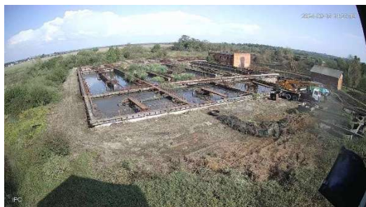
Photo: existing condition, 2026
