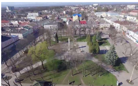
Photo: existing condition
