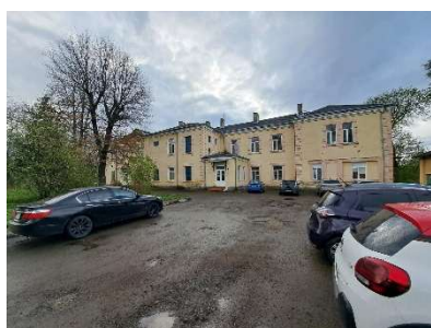
Photo: existing condition, 2026
