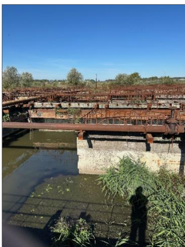
The settling basins, pumps, and other equipment in Stryi's wastewater treatment plant are severely deteriorated.
