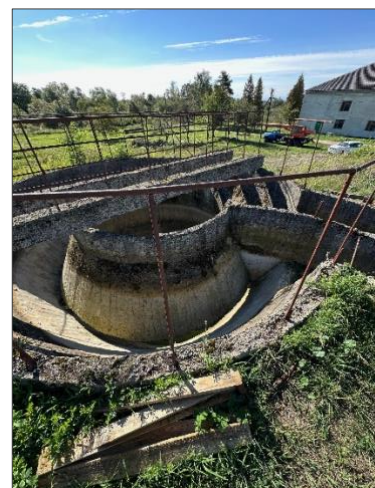
The settling basins, pumps, and other equipment in Stryi's wastewater treatment plant are severely deteriorated.
